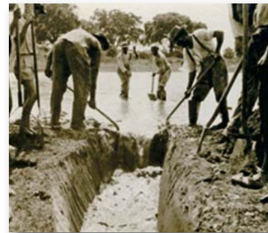
Digging a drainage ditch to reduce mosquitoes
