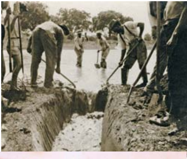
Figure 2: Digging a Drainage Ditch to Reduce Mosquitoes (source: CDC)
