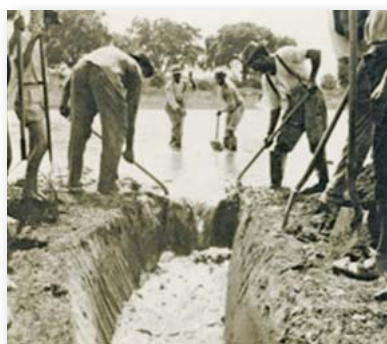
Digging a drainage ditch to reduce mosquitoes
